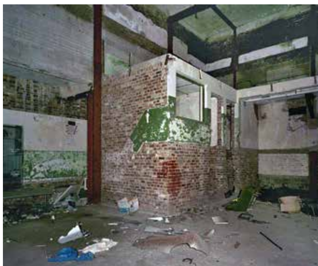
Site of filter room (to the right) in, May 1996.
